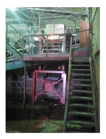
a. The analyzer was installed on a special frame with 11 m height. This frame was placed on a concrete base that has no contact with the metal structures of the conveyor to reduce the vibration that would probably come from the conveyor.
